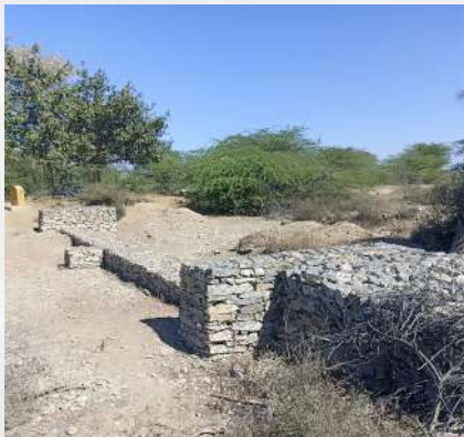
Fig 1: Gabion structure preventing soil erosion.
