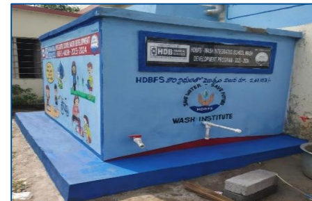
Safe Sanitation Complex, WASH
