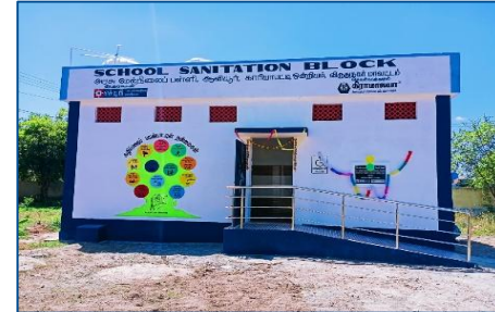
Safe Sanitation Complex, WASH
